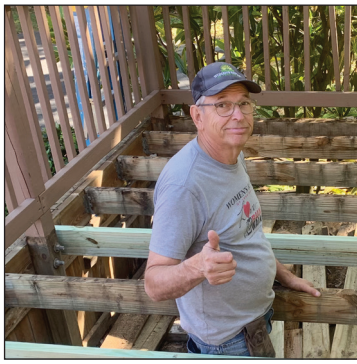
Brian Bogart doing demolition work and prepping porch for project day.
